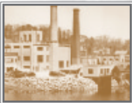
Allen Street plant estimated to be worth $1 million.
