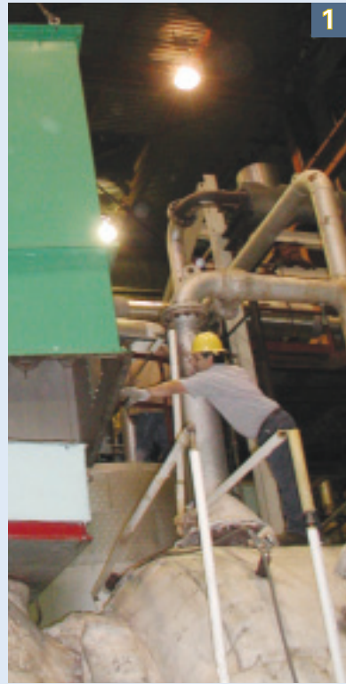
Large sections of air ductwork, piping, insulation, and casings are systematically disassembled before the turbine rotor is finally removed and placed on support stands.
