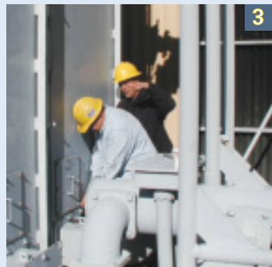
Large sections of air ductwork, piping, insulation, and casings are systematically disassembled before the turbine rotor is finally removed and placed on support stands.
